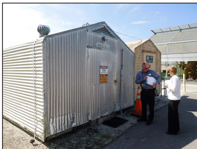
Figure 5.12: Locked metal pesticide storage facility. Credit: UF/IFAS Pesticide Information Office.
